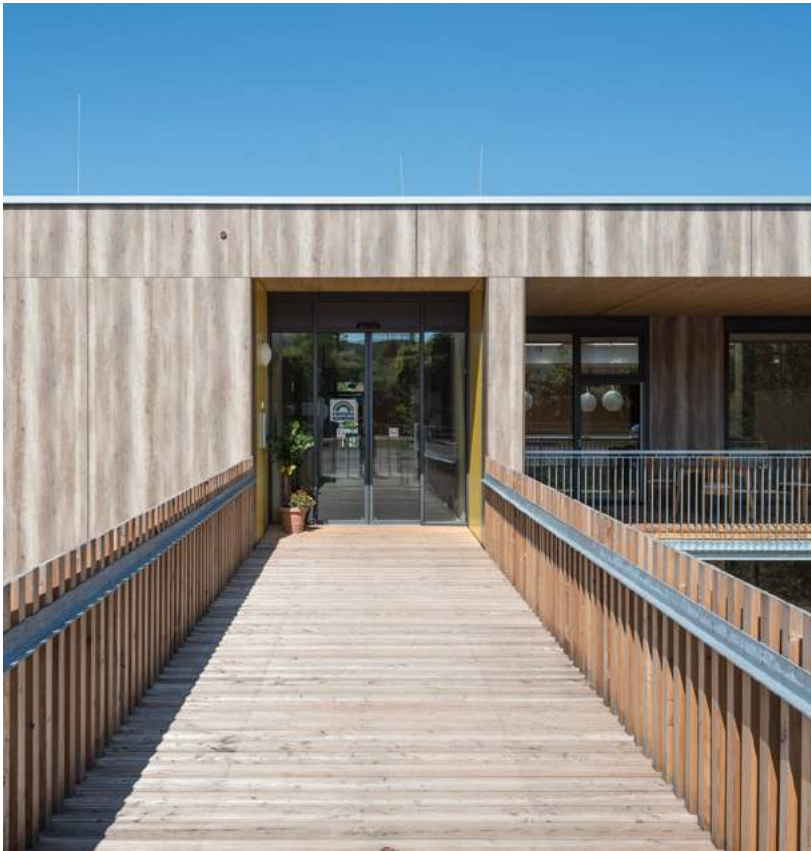
Children's Home Jöhlingen Germany, Walzbachtal
