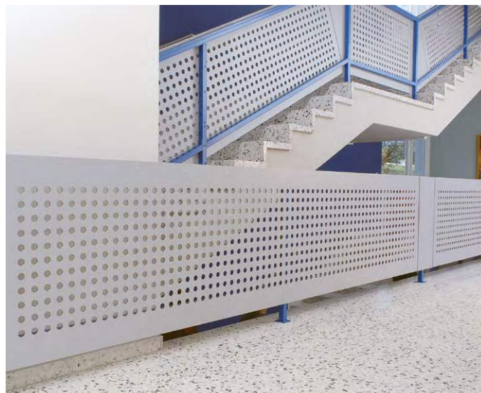
STAIR RAILING - HOLE MILLING
