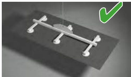
Use lifting system for large-sized panels.
