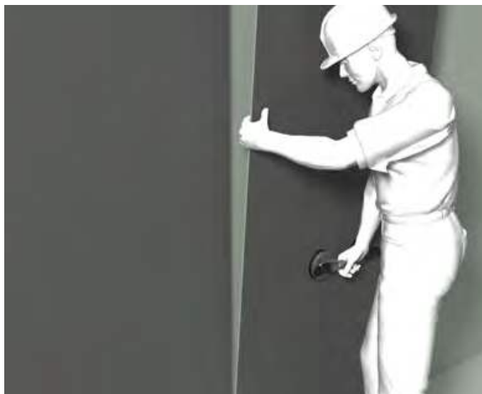
Place panels with suction handles
